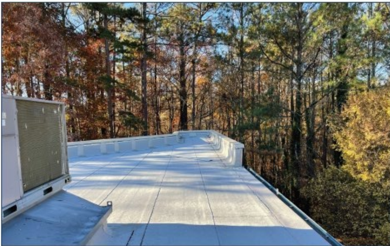
Detail of lower roof section with cap sheet and wall flashing completed
