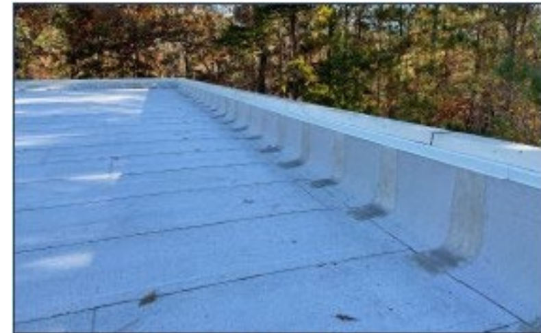
Gym roof section, counter flashing completed
